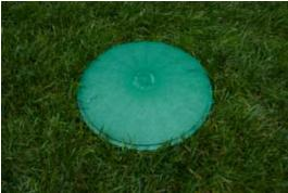
\* A septic tank riser is a concrete or plastic tube that connects to the main manhole (cleanout) of the septic tank, and extends upward, to ground level, thus making the tank easier to access for cleaning/pumping.
